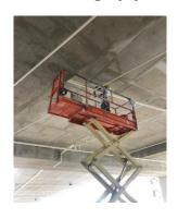
Damaged PVC pipe supports are replaced with metal supports to the existing drainage pipes on the ceiling.
