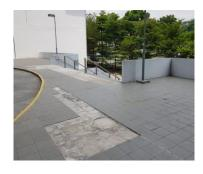
The damaged floor tiles at the roundabout will be replaced with new ceramic tiles.
